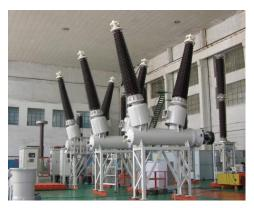
Gas-insulated high voltage switchgear typically use an SF6 gas to minimize arcing when the circuit breaker is activated. Leak testing of the subassemblies and finished product provide confidence that the sufficient pressurized SF6 gas will be contained inside the unit to prolong its functional life. Leak testing also minimizes maintenance and reduces environmental emissions.
